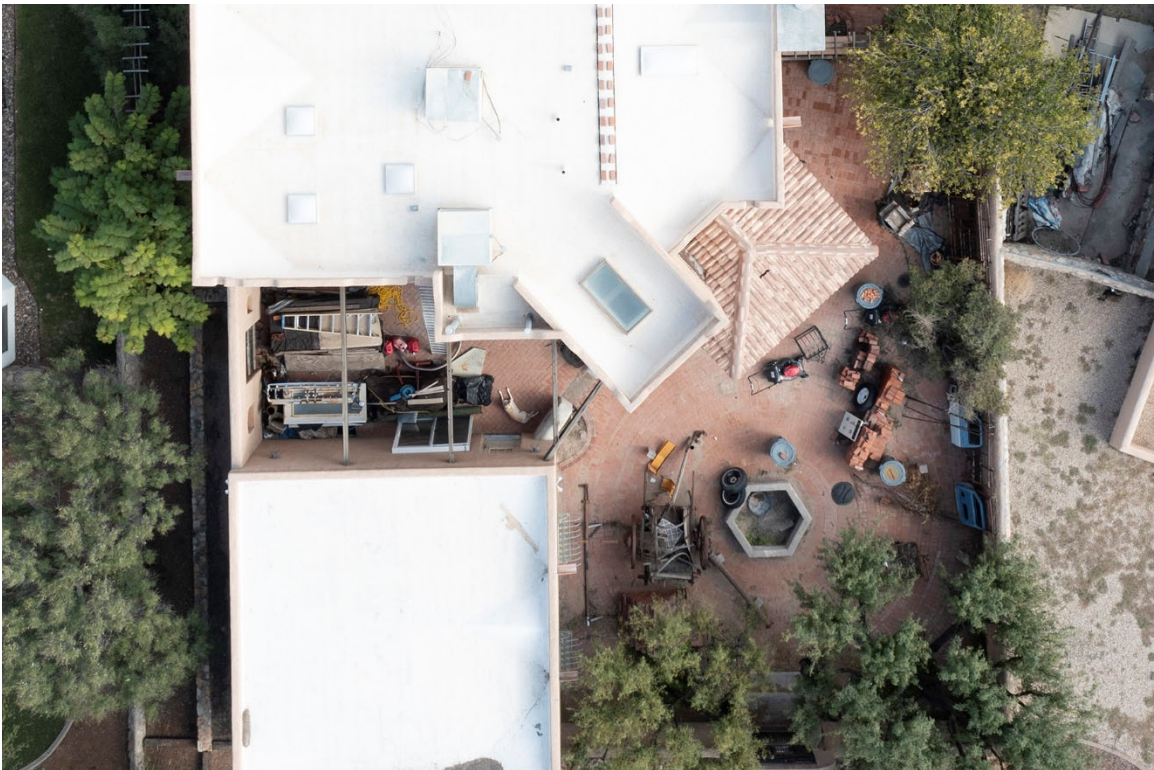
104 Puesta Mirador, Violations of Declaration §§ 11.1 Residential Use, 11.5 Nuisances, 11.9 Garbage , 11.11 Safe Condition
