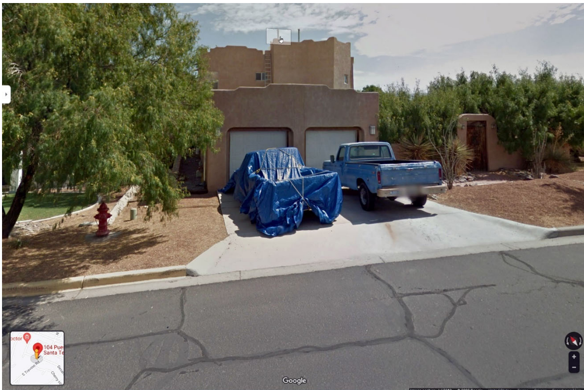
Henry Trost, 104 Puesta Mirador, Violating Declaration § 11.6; Guidelines § 2.1.2
